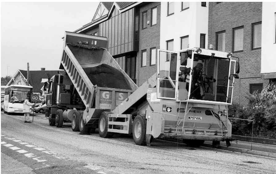
Chipping spreader being loaded
